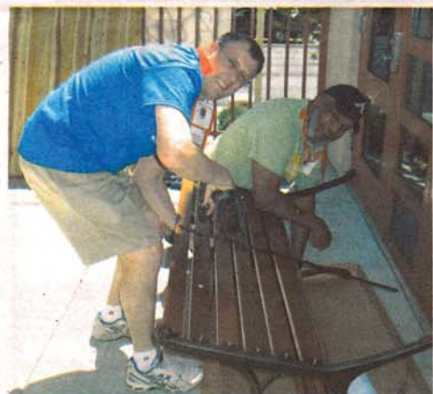
Volunteers building garden bench and wooden fence
